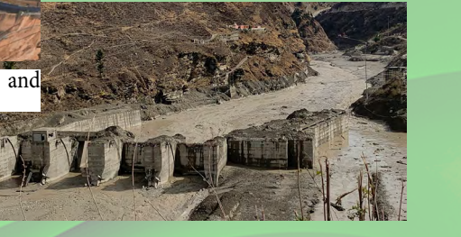
Power Plant Projects gets damaged due to Glaciers Breakoff floods at Uttarakhand.
